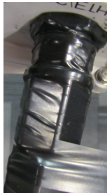
Figure 3.8. Wrapping the Connector with Electrical Tape
